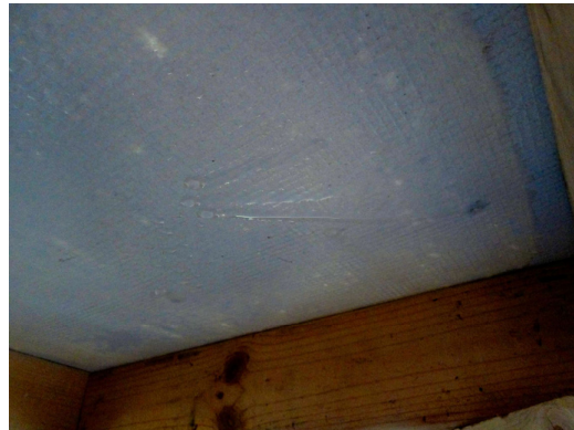
PhotoNo.4 ASTM C1185 – Mockup Specimen Underside Water Droplet Formation Detail
