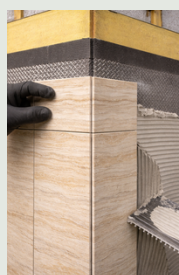
Outside Corner Grouted Corner Joint
